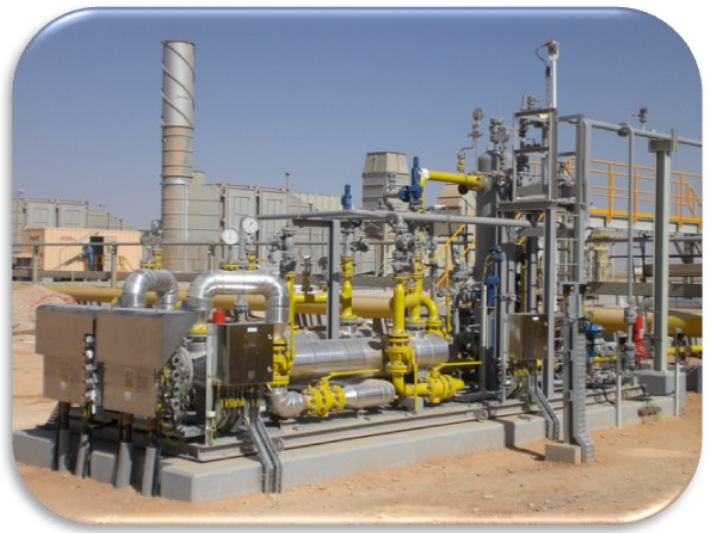
Hydrocyclone skid with control system
