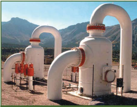
Two Peerless Multi-Cyclone Scrubbers installed at a metering station in western Canada. Typical natural gas flow through these 2000mm diameter vessels is 2.5 billion standard cubic feet per day.
