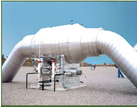
A 2500mm diameter Peerless Swirl Tube Separator installed in a gas gathering system. Typical flow is 3 billion standard cubic feet of gas per day.
