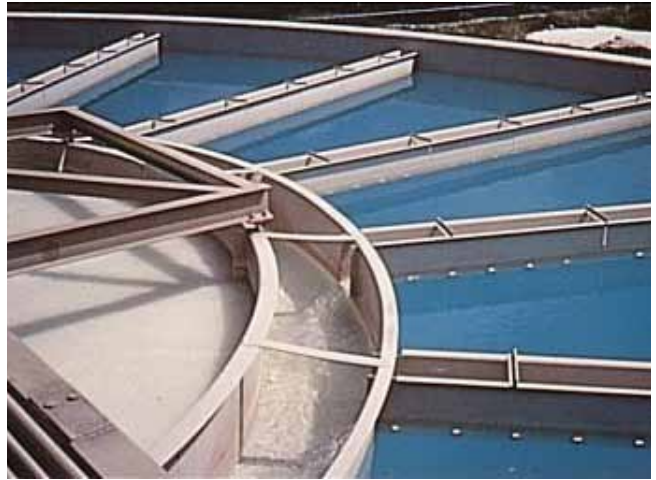
(Top) Reactor Clarifier (Bottom) Thickeners
