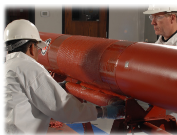
Wrap barrier fabric on pipeline.
